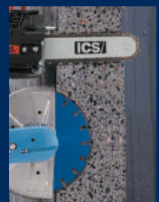
4. Finish off corners and remaining depth with diamond chainsaw.
